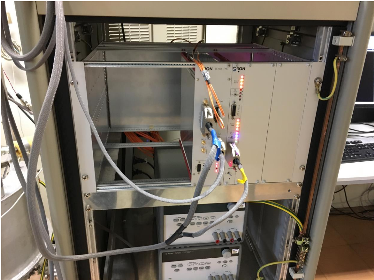
Fig. 4.3: DEMUX FMC-II 10 under test.
