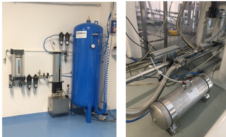
Figure 4: Left: The filtering system for the air used for venting. Right: A small stainless-steel tank is placed close to the clean tent to have clean dry air available for the optics cleaning, if needed
