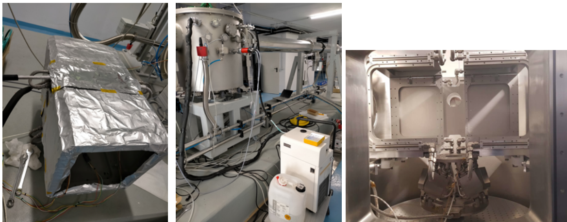
Figure 6: Left: the thermal box cover with UHV Al foil. Centre: the chiller connected to the thermal box via feedthroughs. Right: the thermal box inside the MM Chamber [PR#35]
