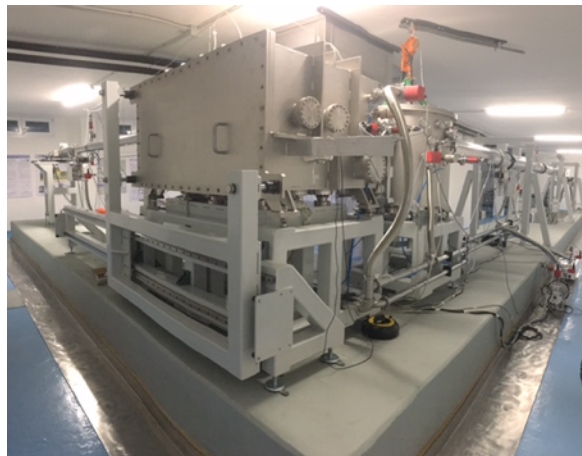
Figure 2: The BEaTriX vacuum system positioned over the isolated foundations
